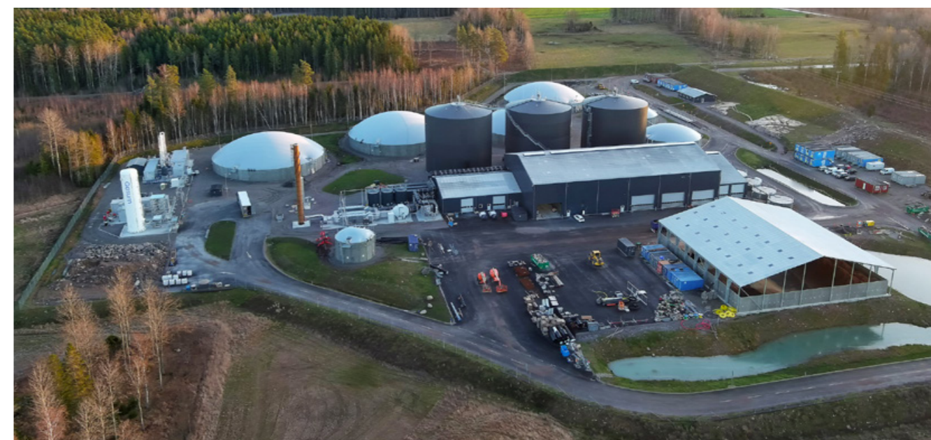
Gasum's new plant in Götene, which will produce 120 GWh of liquefied biogas per year, mainly from manure.
